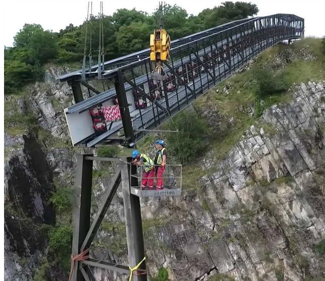
Figure 2: Dizzying heights the technicians mount the suspended elements of the conveyor to the steel structure. Cranes were used to exactly manoeuvre the assembly
