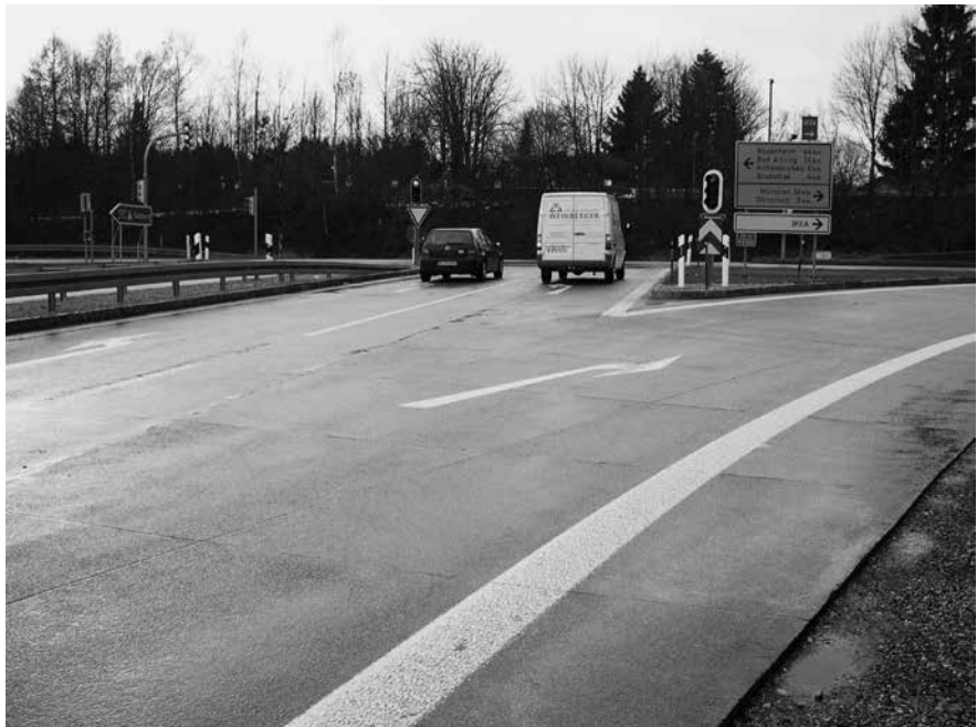
Fig. V-54: Whitertopping concrete pavement for a motorway connection
