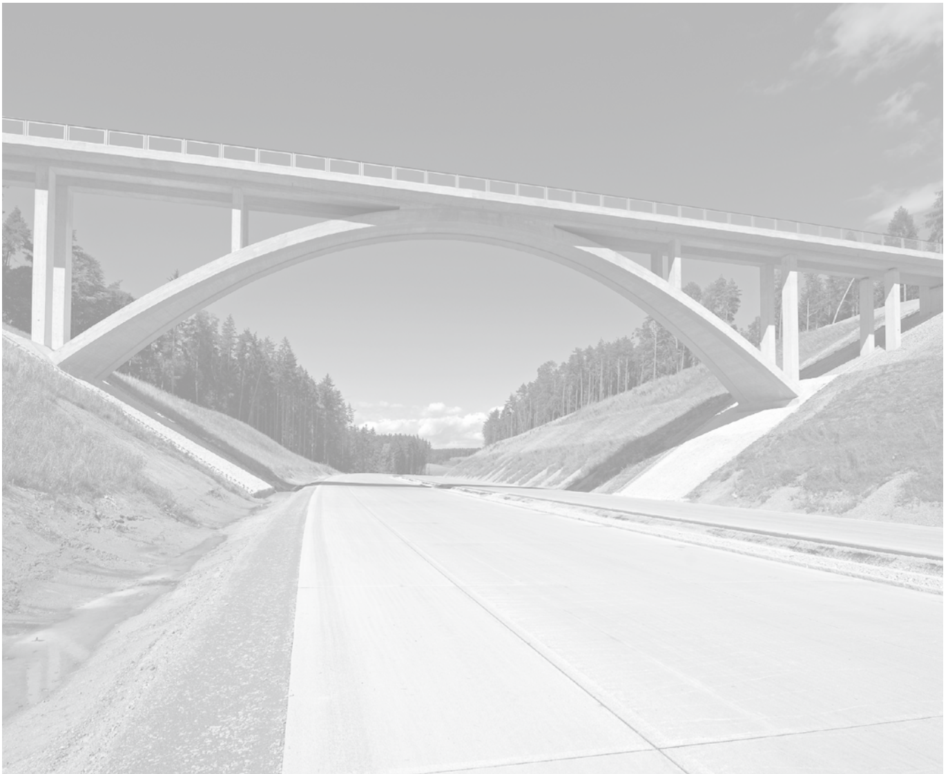
B15n between Schierling and Neufahrn: Concrete surfacing of the first 22 km construction section
