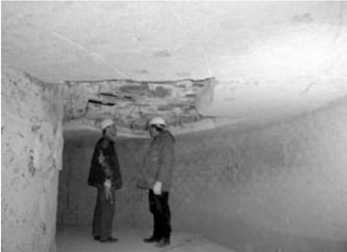
Fig. I-14: Cyclone ceiling segment that has fallen out
