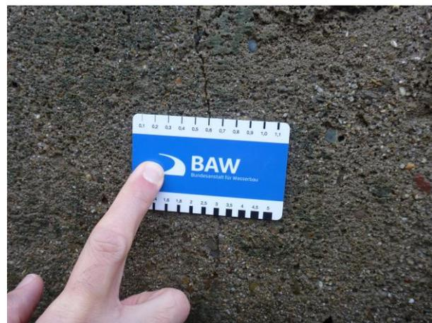
**Figure 6.** Vertical crack in wall of lock 1 with a crack width of up to 0.6 mm.
