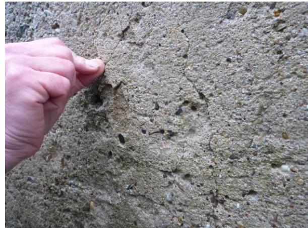
**Figure 4.** Concrete surface damaged by freeze-thaw attack at lock 3 can be peeled off by hand.
