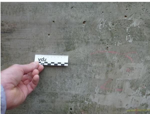
**Figure 5.** After 11 years of service life lock 4 showed the least damaged concrete surfaces.
