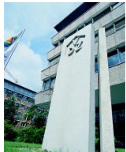
Fig. 1: On 1 June 1956 the Research Institute started operations in the newly erected VDZ building. Since 1998 the concrete steles stand in front of the newly designed entrance hall.
